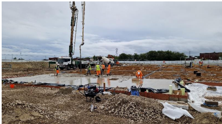
Concrete to ground floor slab
