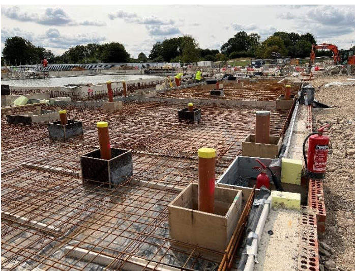
Ground Floor Preparation
