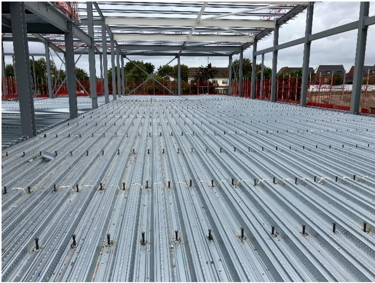
Metal deck to upper floors
