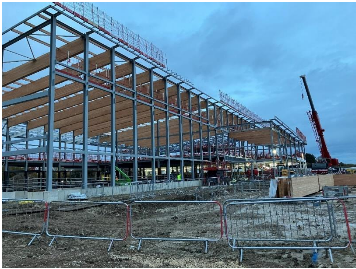
Structural Frame and Glulam beams.
