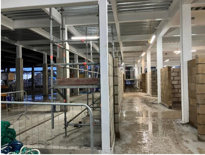
Blockwork to Ground Floor
