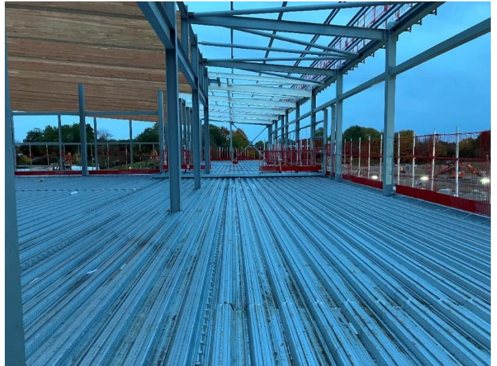
Upper floor decking
