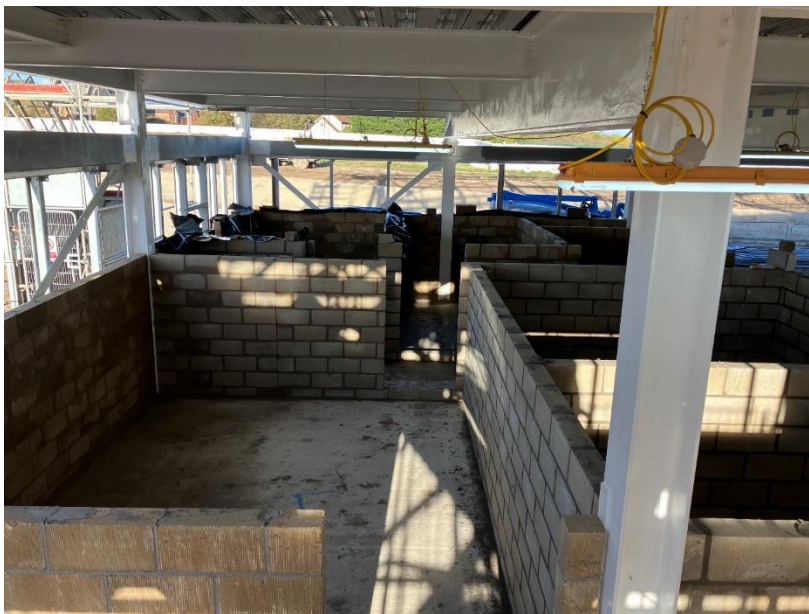
Blockwork to ground floor
