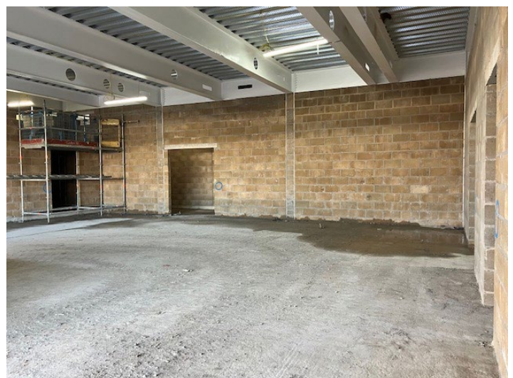
Ground Floor Blockwork
